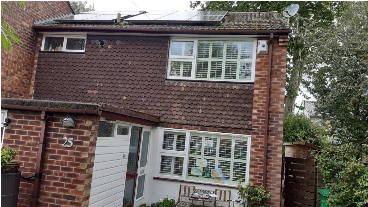
Front view of No.25 Hampton Road
