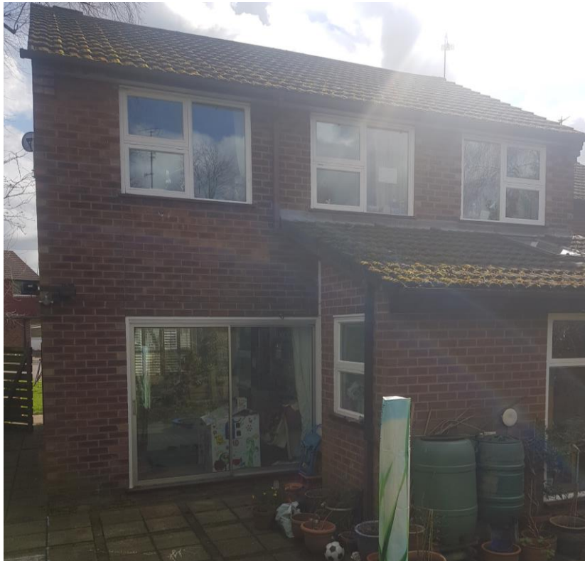
Rear view of No.25 Hampton Road
