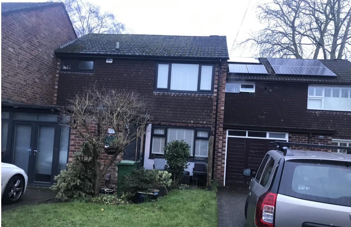
Front view of No's 23 and 25 Hampton Road
